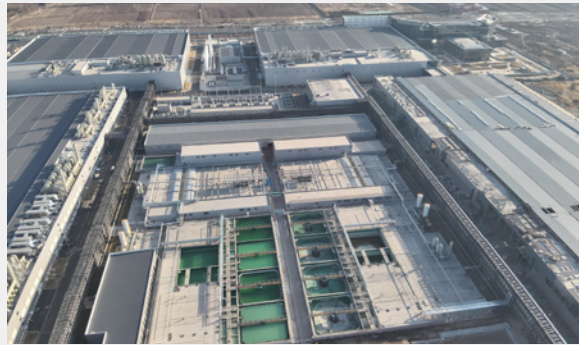
Wastewater Treatment System
