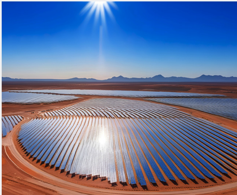
UAE Abu Dhabi Ajban PV3 Photovoltaic Project
